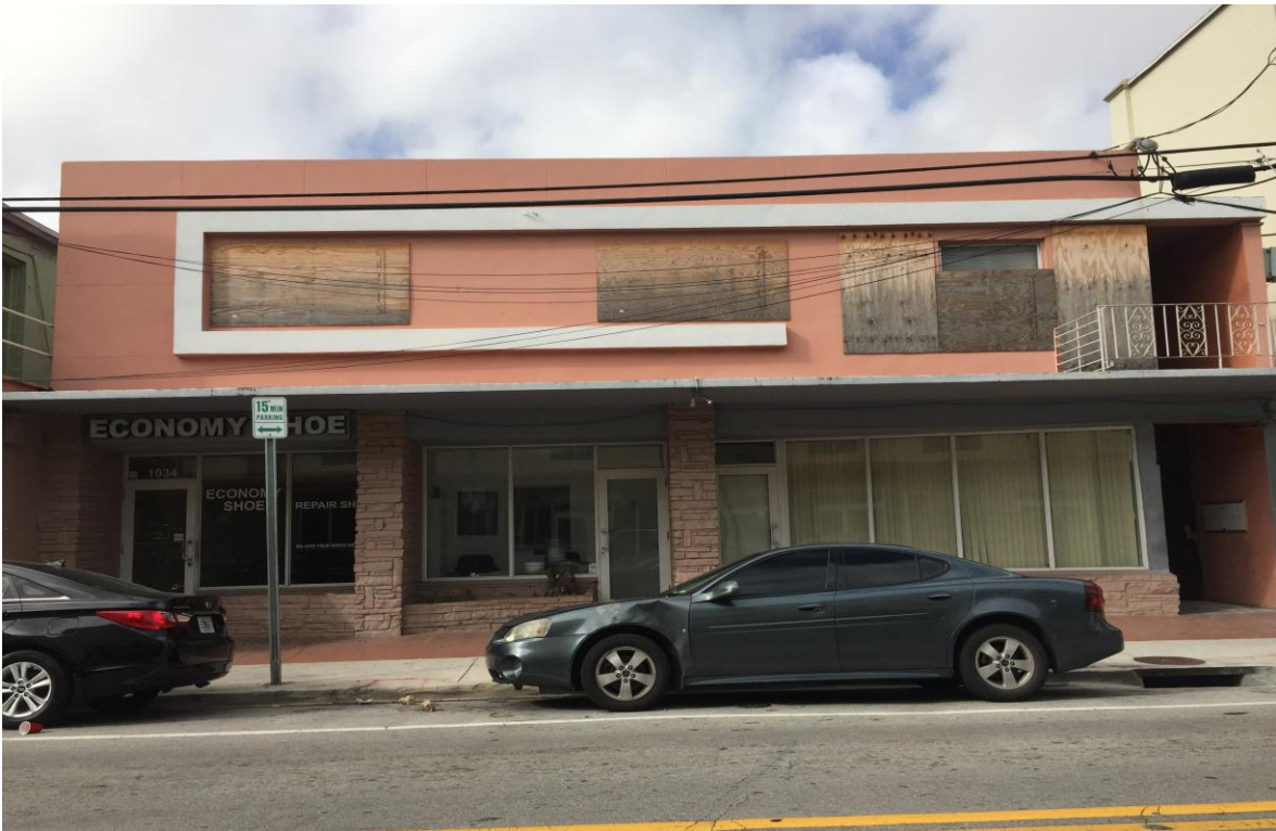
1034 NW 3 rd Avenue: Main façade (2015).
